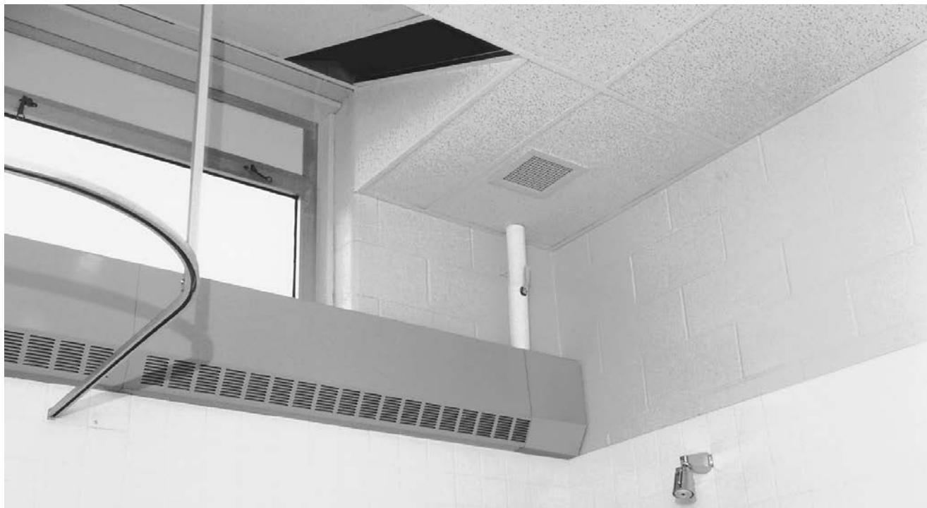
8", 11", 14", 20" and 24" high Versa-Line enclosures can be inverted using standard brackets and ball bearing hangers.
